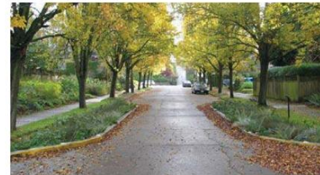
Bulb-outs with bioswales can be a natural extension of the streetscape environment.
