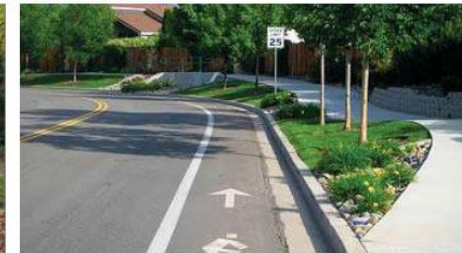
Striping and markings clearly define the bike lane.
