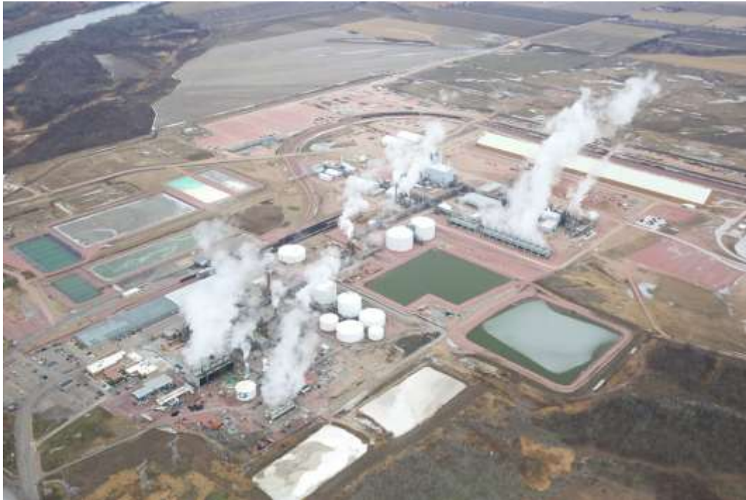
CF Industries plant facility. Image source: MessengerNews.net
